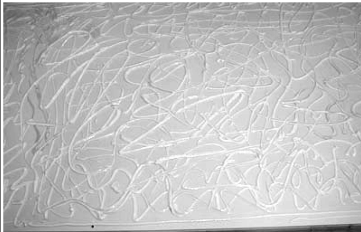
Figure 1: Typical Green Glue Random Application Pattern (photo by client)
