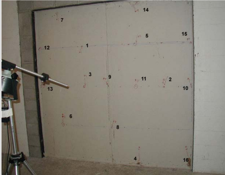
Figure 2: Finished Specimen (fastener at numbered location 1 intentionally short-circuits the resilient channel; numbered locations 2-16 for subsequent testing)
