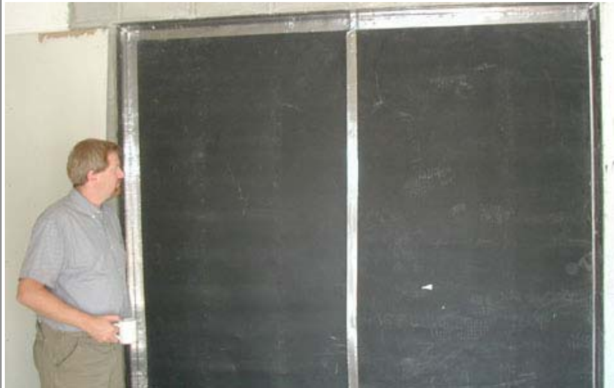
Figure 1: Mass-Loaded Vinyl Sheets on Unfinished Wall Assembly Interior
