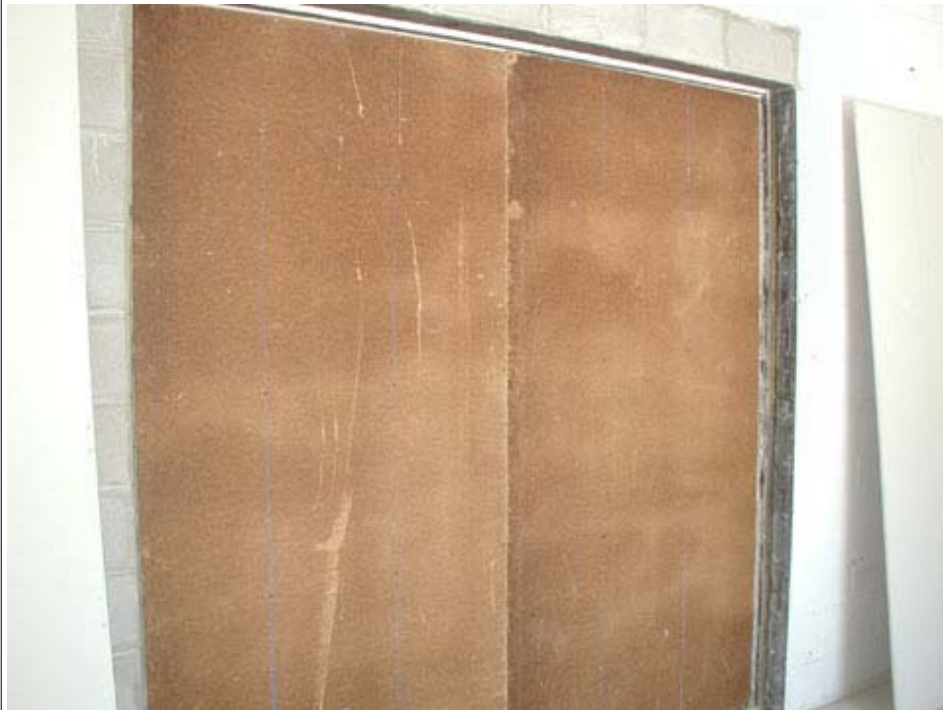
Figure 1: Installed Base Layer of Sound-Deadening Fiberboard
